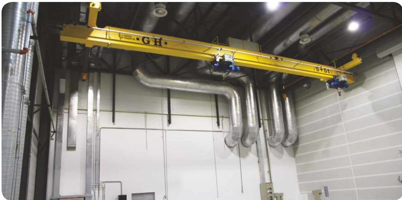
SINGLE GIRDER: CAPACITY UP TO 20+20t.
